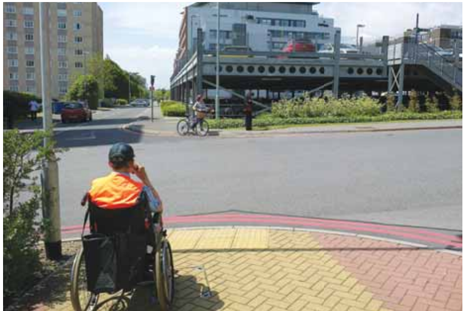
Pedestrian waiting at a crossing with no corresponding dropped kerb on the opposite side of the road
